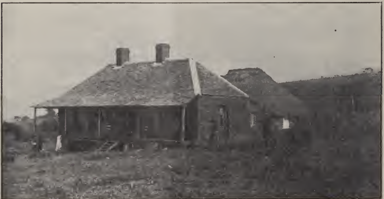
The Teachers' Residence at Mt. Silinda
